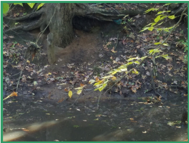
More advanced erosion.
